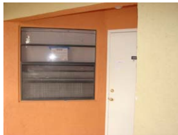
Front Door Entry
