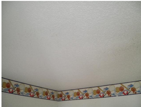
41. Interior Room Ceiling
