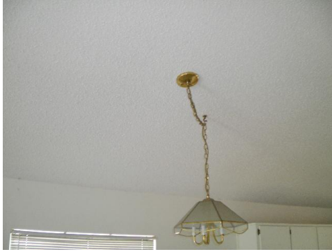
26. Interior View Ceiling
