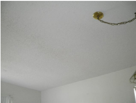
31. Interior View Ceiling
