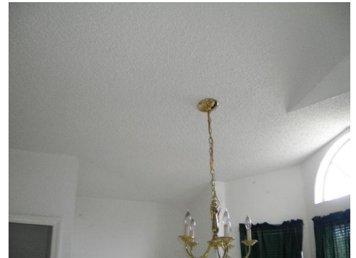
42. Interior View Ceiling
